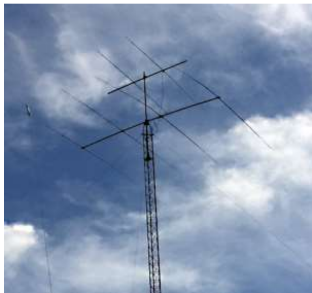
Fig. 2 - W5RRR 20m/15m Yagi- note the 15m Yagi on top w/only 2 remaining elements
